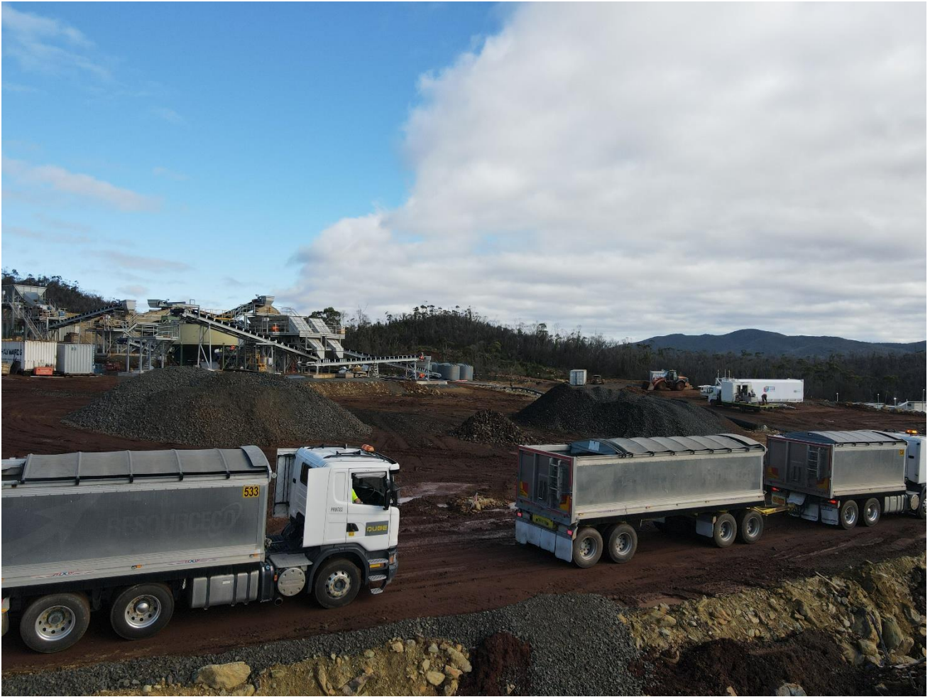
Figure 2 | Qube trucks on site for test run and site inductions.
