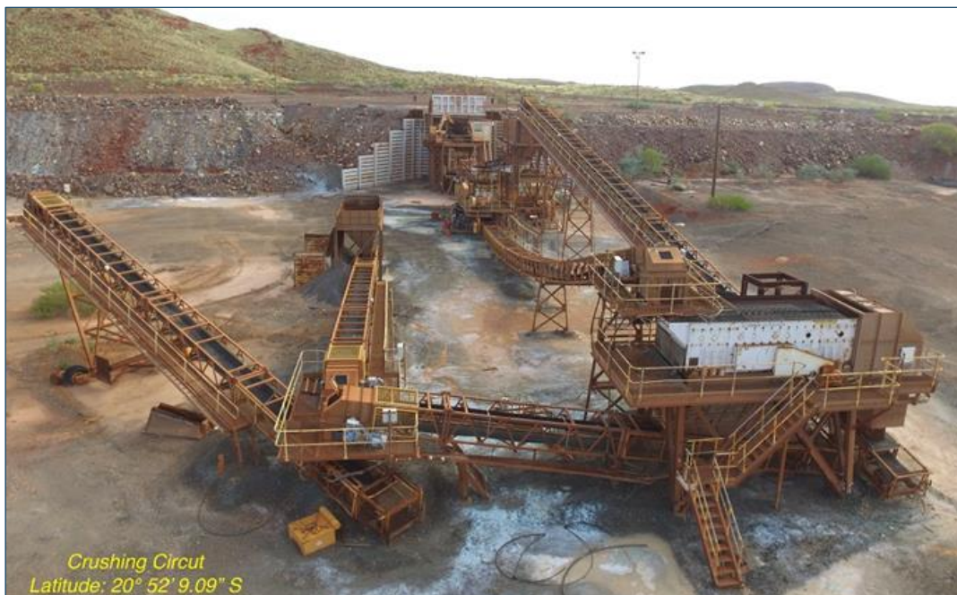
Figure 2: The Whim Creek crushing circuit to be refurbished with an integrated sorting circuit
