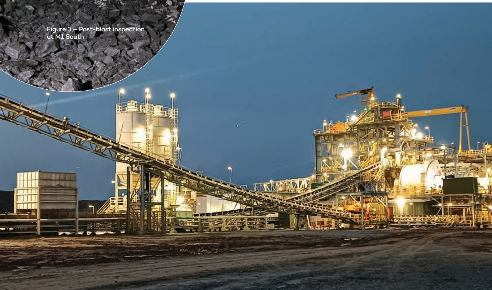
Figure 4 – Sanbrado process plant
