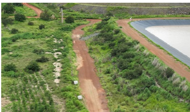
Progressive rehabilitation around Water Storage Facility, Sanbrado
