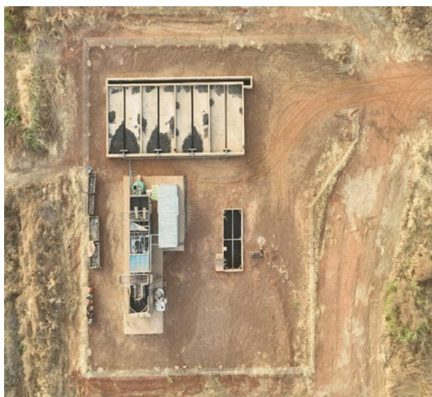
Kiaka wastewater treatment plant
