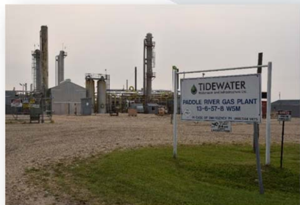
Figure 1 - Tidewater Gas Plant
