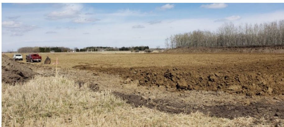
Figure 2 - Multi-well and facilities pad under construction
