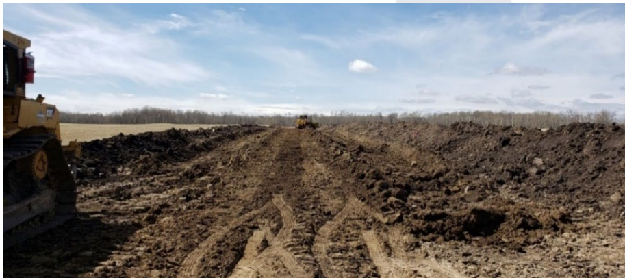
Figure 1 - Access Road under construction
