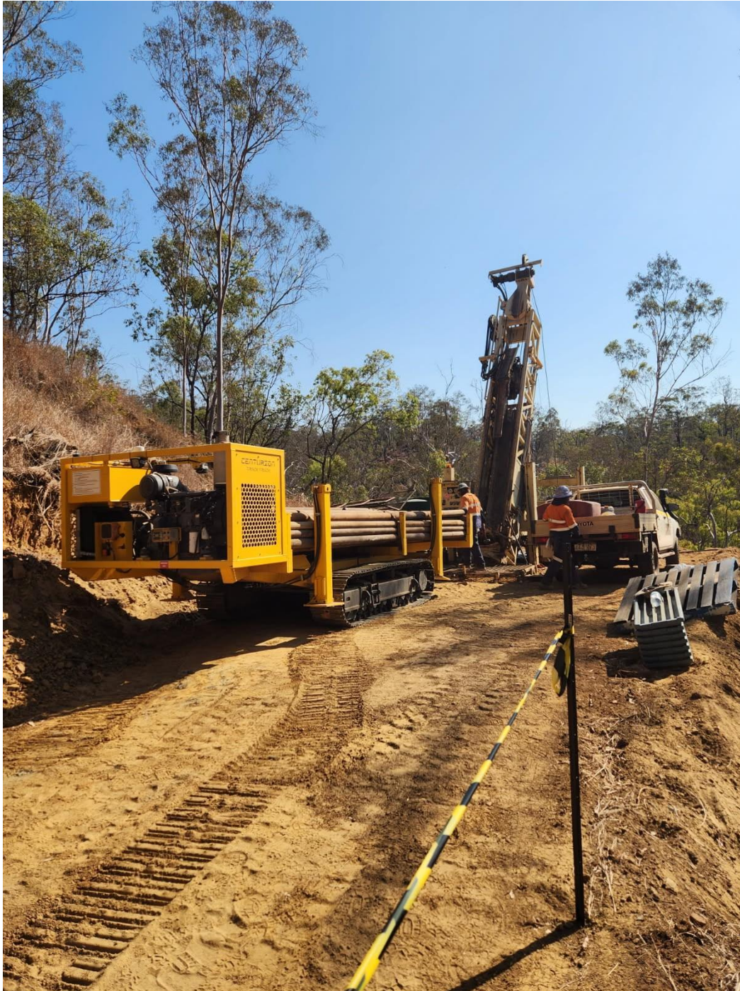
Figure 1: Core-drilling program commencing in the Specimen Hill Project, Central Queensland.
