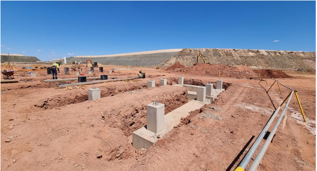
Figure 2: Stage 1 Development: Construction of the Concentrator – early photo of the Flotation Concentrator concrete foundations
