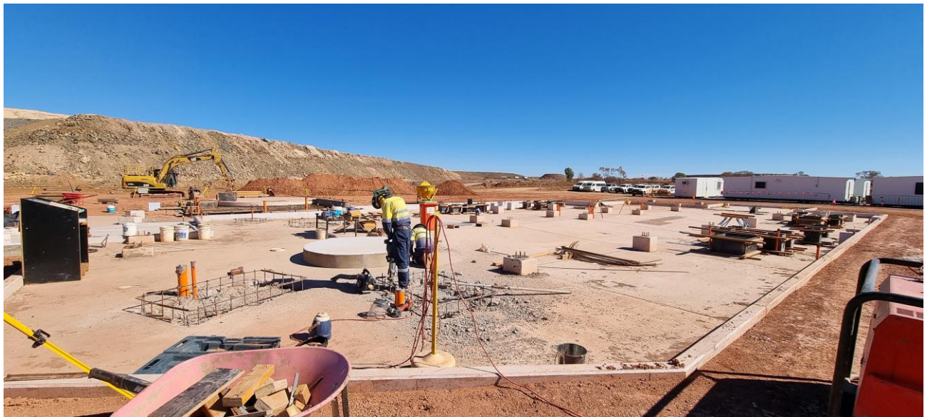
Figure 3: Stage 1 Development: Construction of the Concentrator – concreting of the Flotation Concentrator concrete foundations Progressing to Plan
