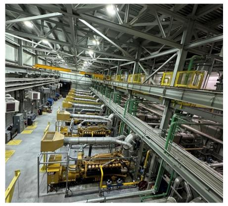
Image 6. Natural gas generators housed within the power station.
