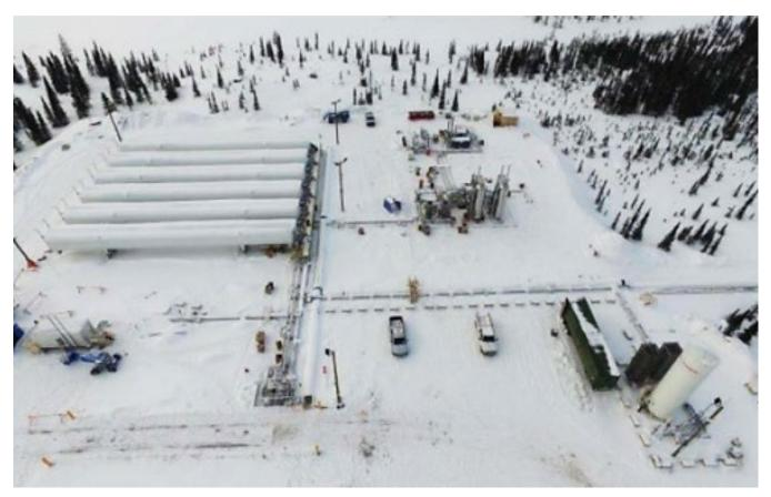
Image 7. LNG storage tanks on site at Renard.
