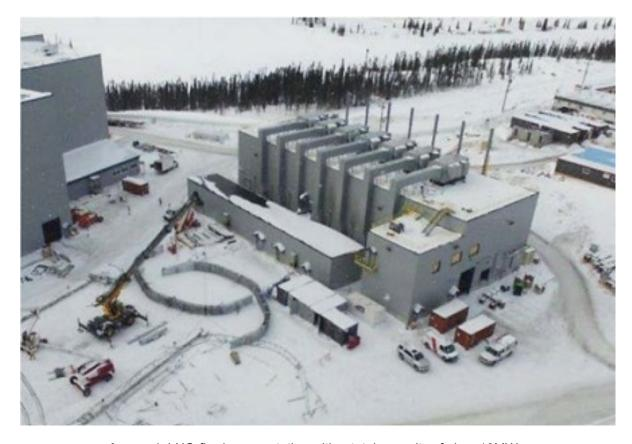
Image 4. LNG-fired power station with a total capacity of circa 16MW.
