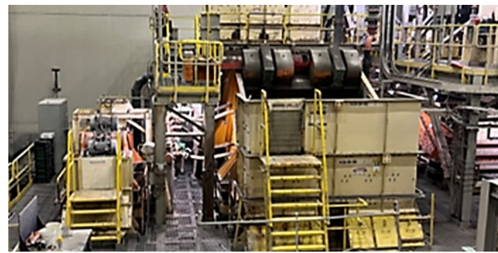
Figure 5. Inside the Processing Plant
