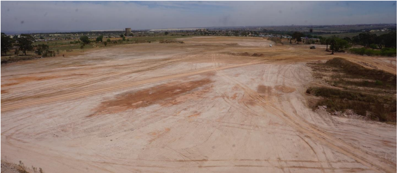
Image 3: Pit 1 has been completely backfilled, removing illegal miner access to the historical underground mine works and delivering on a key milestone of the Government Directive.
