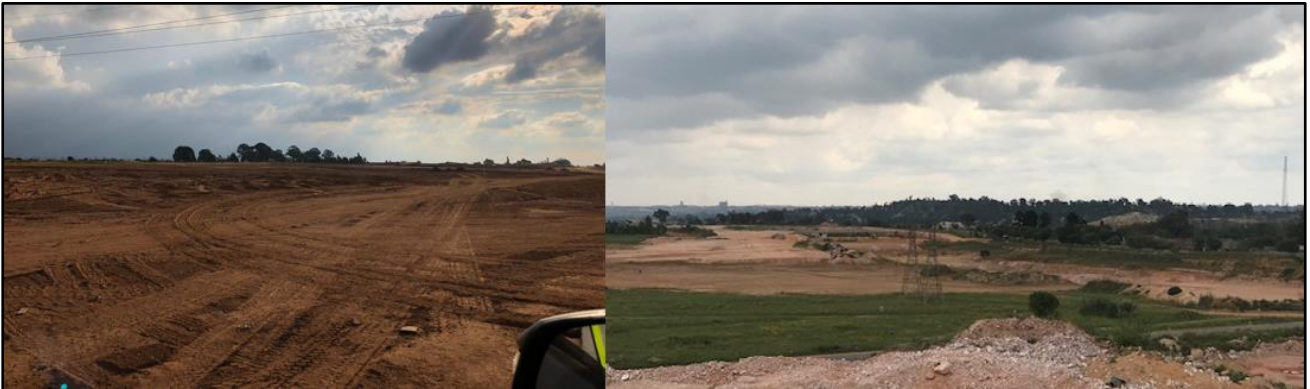
Image 4: Pit 2's rehabilitation completed during the quarter
