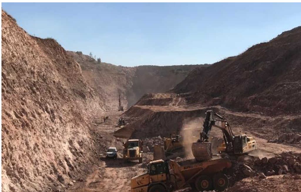
Image 1: The narrowing of Pit 3 as it nears completion in June 2019.
