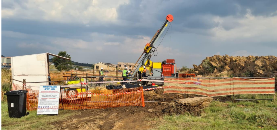
Image 1: Diamond drill in operation at the WBP.
